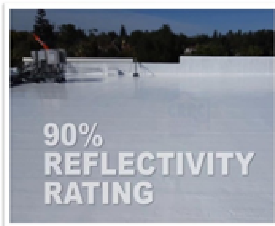
Cool Roof Coating Applied
