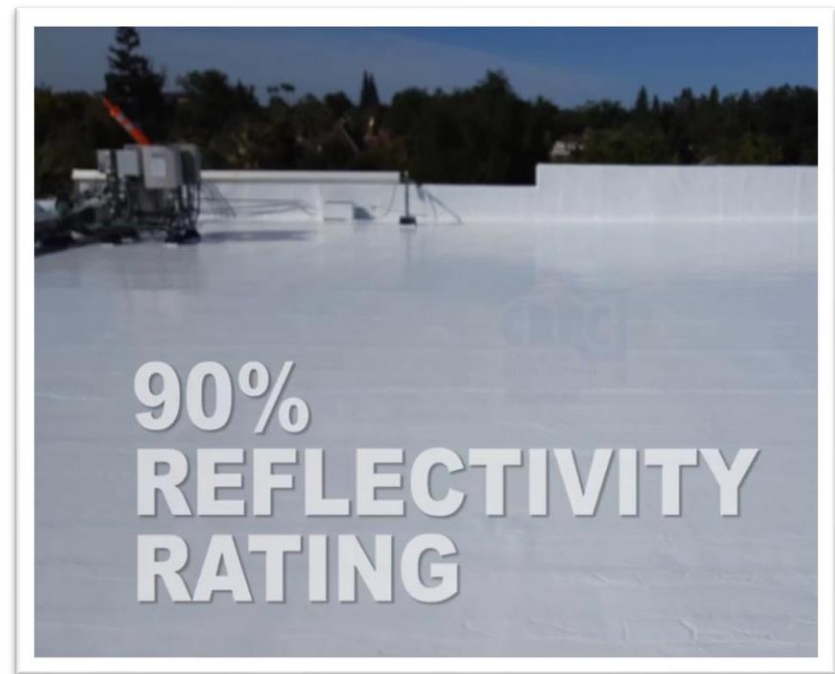
Cool Roof Coating Applied
