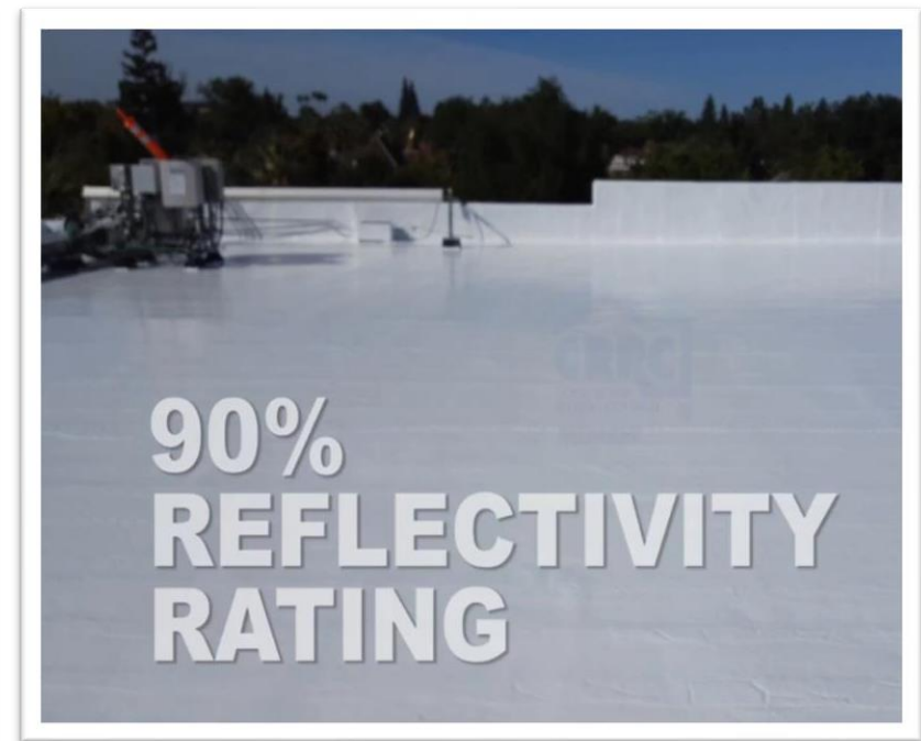
Cool Roof Coating Applied
